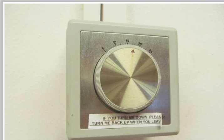
Simple sign from another Oxfordshire village hall
