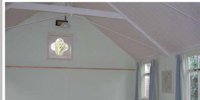
Britwell Salome Village Hall completed internal wall insulation
