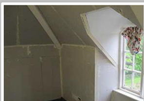
Installation of insulation backed plasterboard
