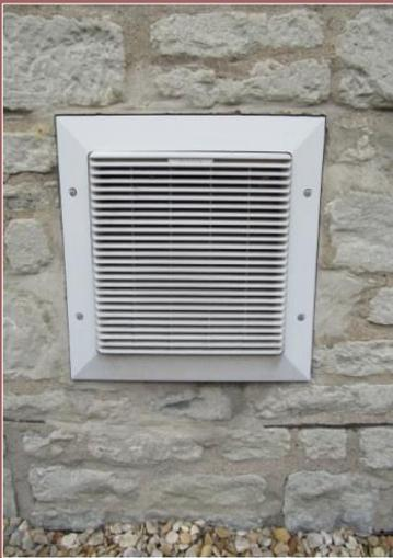
If fridges and freezers are on an external wall, warm air can be extracted directly outside
